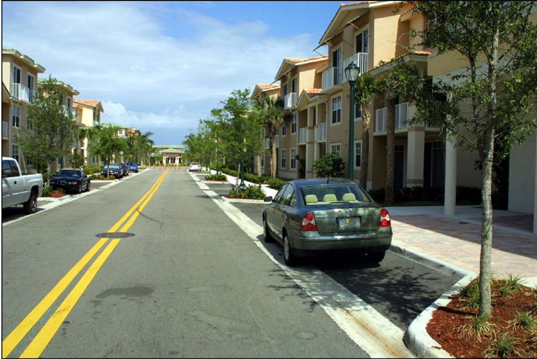
Valley gutters with bulbouts and parking
